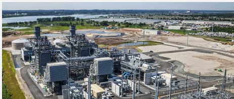
CPV's existing Woodbridge Energy Center
