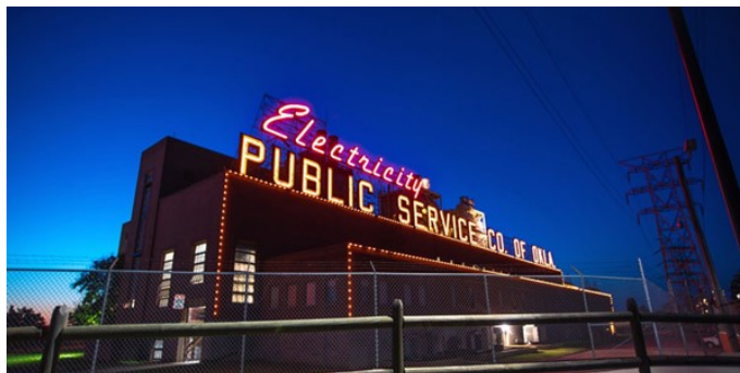
Tulsa Power Station | Public Service Company of Oklahoma
